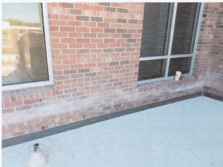
Completed Repair Above Corridor 126 and Classroom 128 Prior to Cleaning
